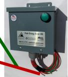
(Two red wires from the Peak Energy Saver connect to the dedicated breaker installed in the main breaker box.)
